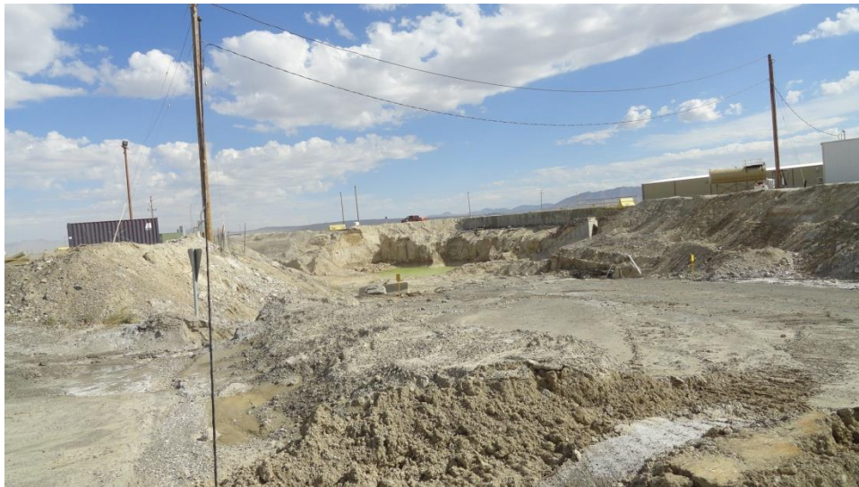
Figure 1. Old Rollover Facility Demolition Area
